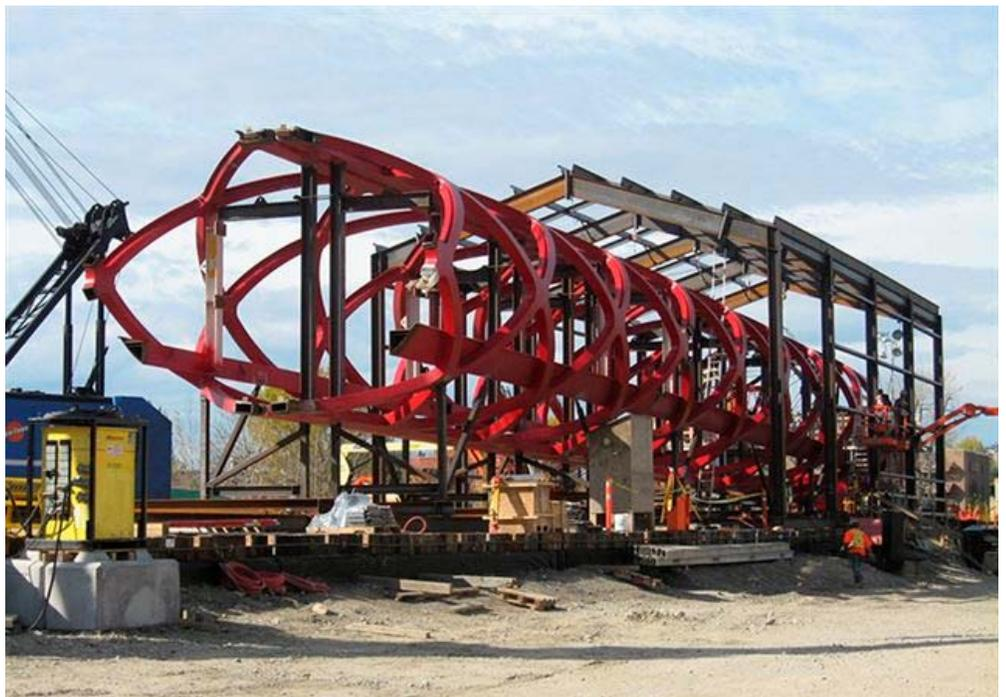
**THE FIRST SIX HALF MODULES ASSEMBLED IN THE WELDING SHELTER**
